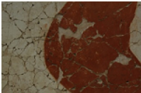
(a) Area with cracks
